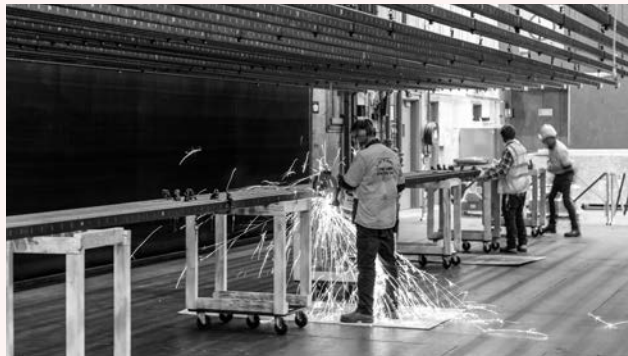
On the State Theatre stage, taking apart the old flying system equipment. Photo credit: Mark Gambino.
