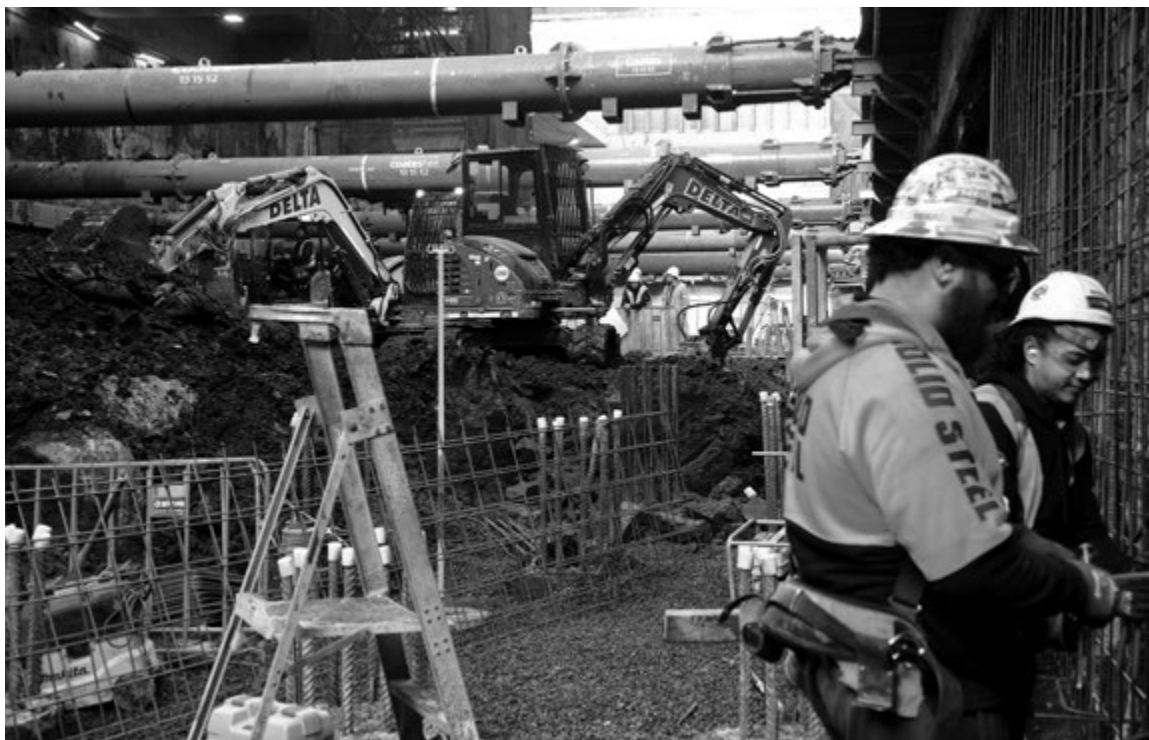
The horizontal supports, called “walers”, are designed to provide extra support as we expand the existing retaining wall of the building. Credit: HiVis Photography, courtesy Development Victoria.
