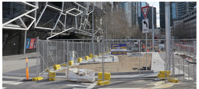
Progress on Stage 2 of Southbank Boulevard.
