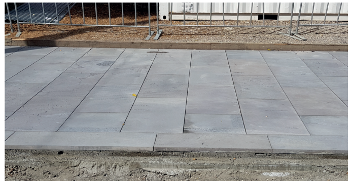
Bluestone pavement currently under construction on Southbank Boulevard
