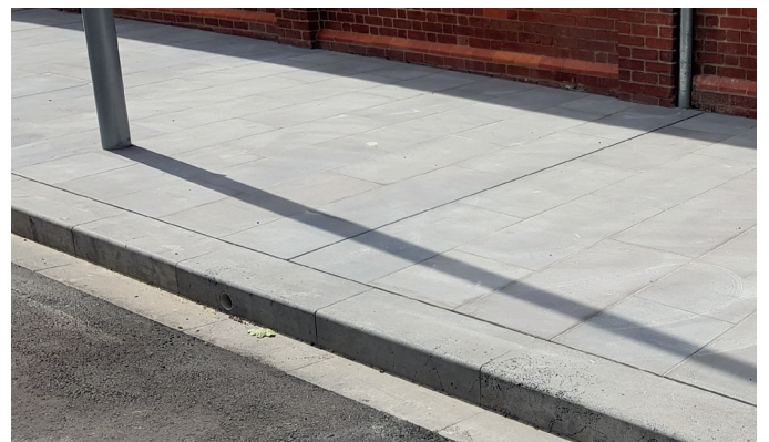
Completed bluestone pavement on Dodds Street.
